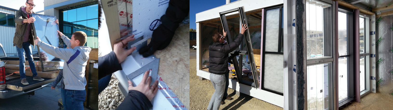
(left to right): Manko generated donated much of the aluminum frame components and all of the glass used in the student prototypes – Nick Nelson and Tyler Countess pick up part of the order produced for them after they specified it to Manko; as part of the process, students learned to properly install glazed curtain walls; Cameron Marshall places his group's frame into the test enclosure; three of the curtain wall prototypes seen from the interior of the test enclosure.
