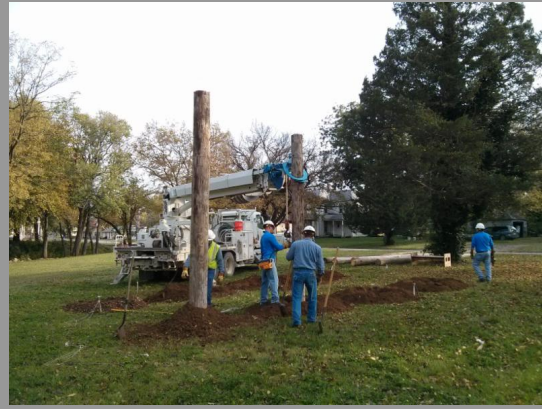
Photo of pavilion columns being set, courtesy of Gabbard.
