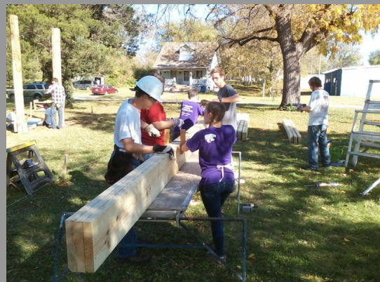
Students fashion built-up beams for roof girders. In
